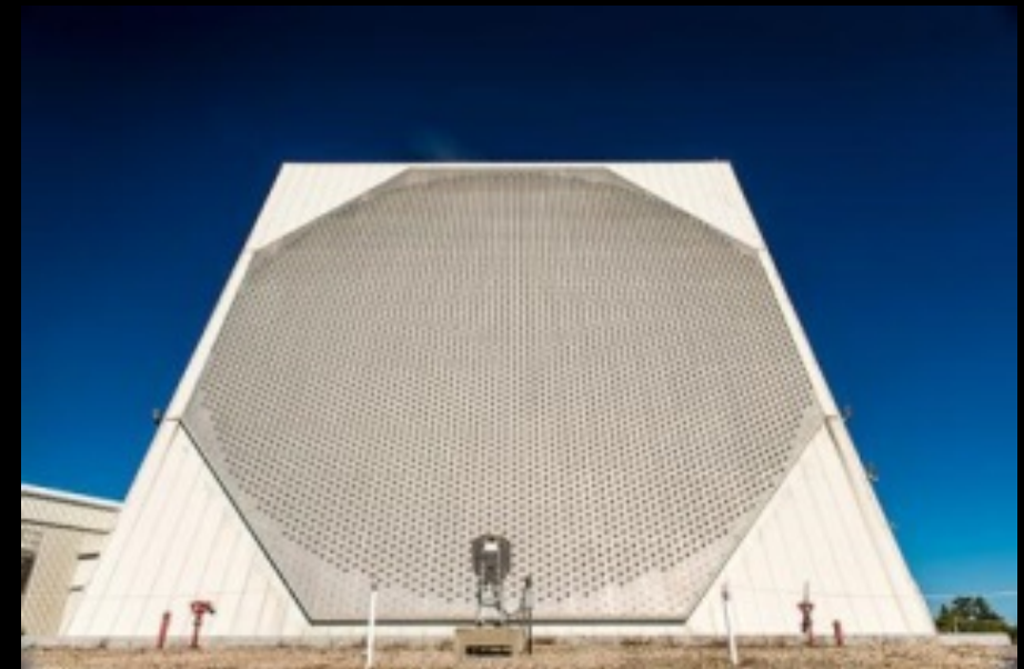
Upgrade Early Warning Radar Raytheon
